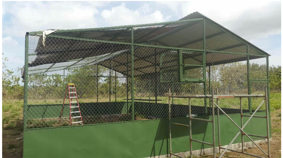
First HTFF aviary construction completed in 2015
